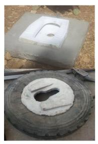
**2. Small Oval Slab:** This option offers households a latrine slab at a very low price. It is designed to be used with a wooden slab. Households would plaster the rest of the wooden slab with mud once they have installed the small slab. Besides its affordability, the slab is easy to wash without spoiling the wood. It also has very good drainage, and it is easy to cover the hole to protect flies.
