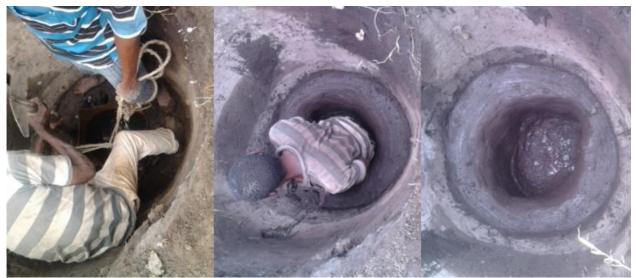
Figure 4: soil cement mixture pit lining
